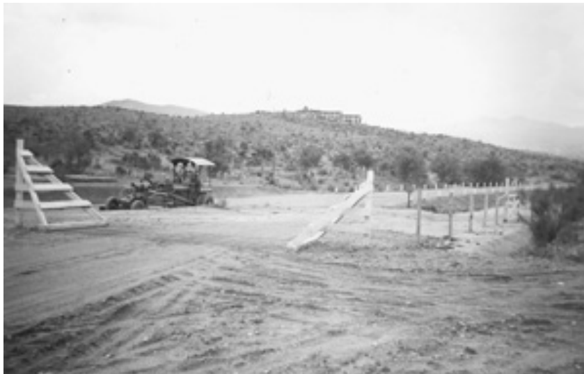
Cattle guard along Highway 82, under construction by workers of the Federal Emergency Relief Administration, 1935. Arizona State Library, Archives and Public Records, History and Archives Division.
