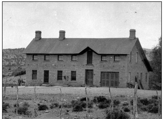
Fort Rock Ranch, Yavapai County, 1913. Arizona State Library, Archives and Public Records, History and Archives Division.
