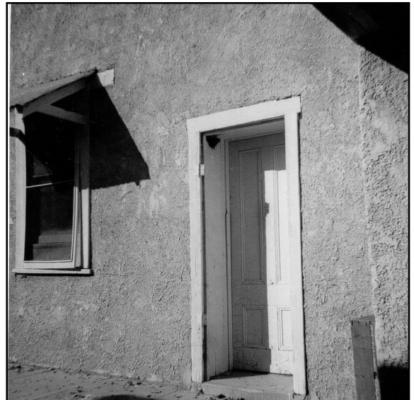
Door in the adobe wall of the Empire Ranch house. SHPO photo collection.
