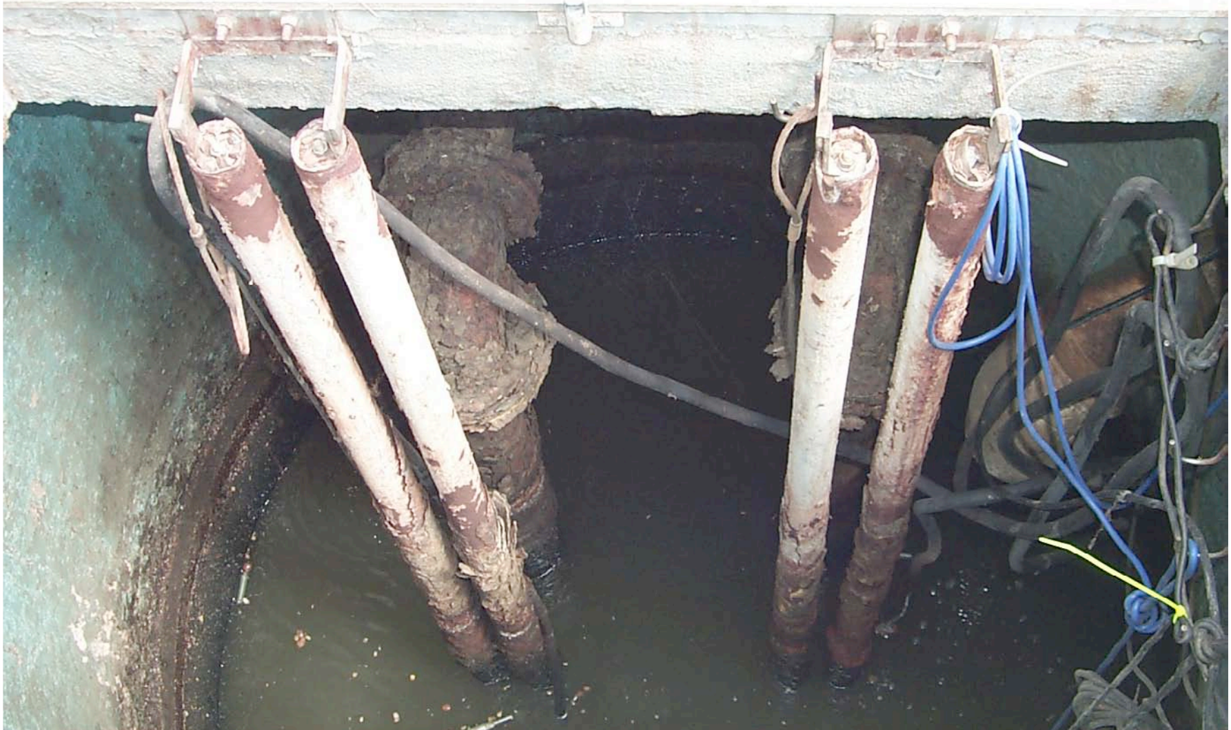
Buckskin - Lift Station before Construction Contract 68.5k SLIF Completion Spring 2010
